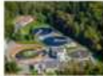
Water treatment & distribution
